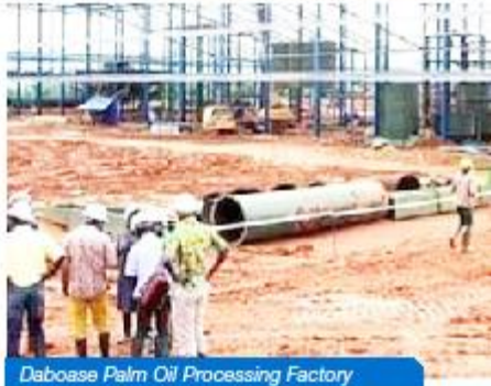
Daboase Palm Oil Processing Factory
